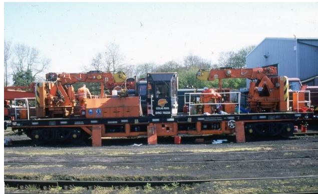
Colas Track Crane also in April 2016
